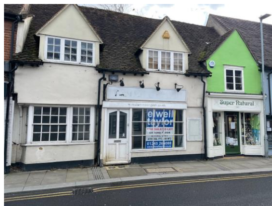
14 High Street in 2023, prior to installation of new shopfront.
