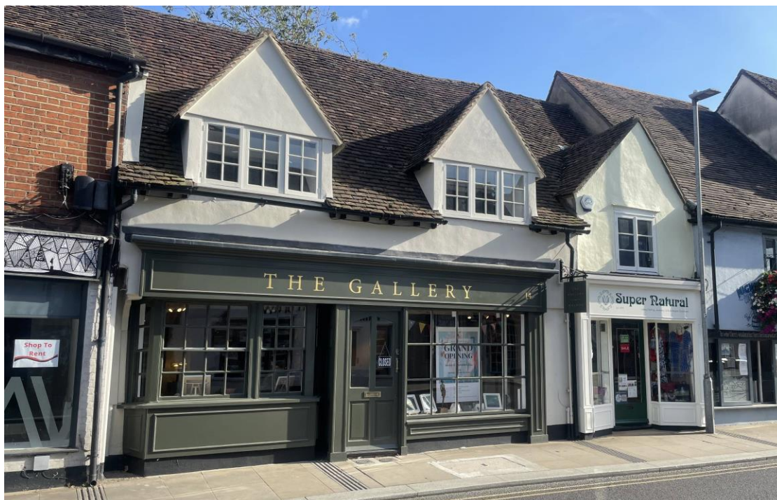
14 High Street in August 2024, with new shopfront.
